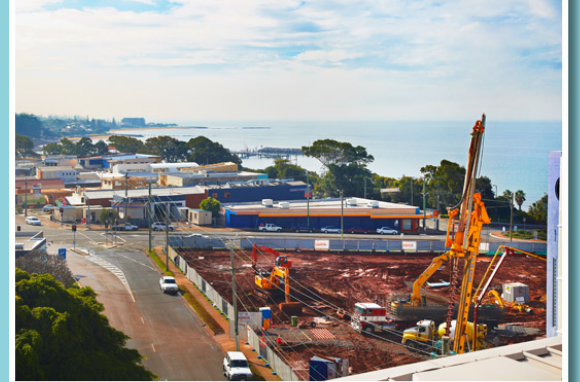
Construction begins! June 2009
